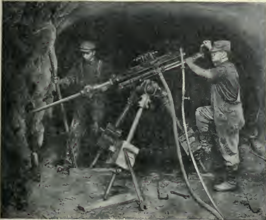
DRILLING SIDE-HOLES FOR WIDENING.
